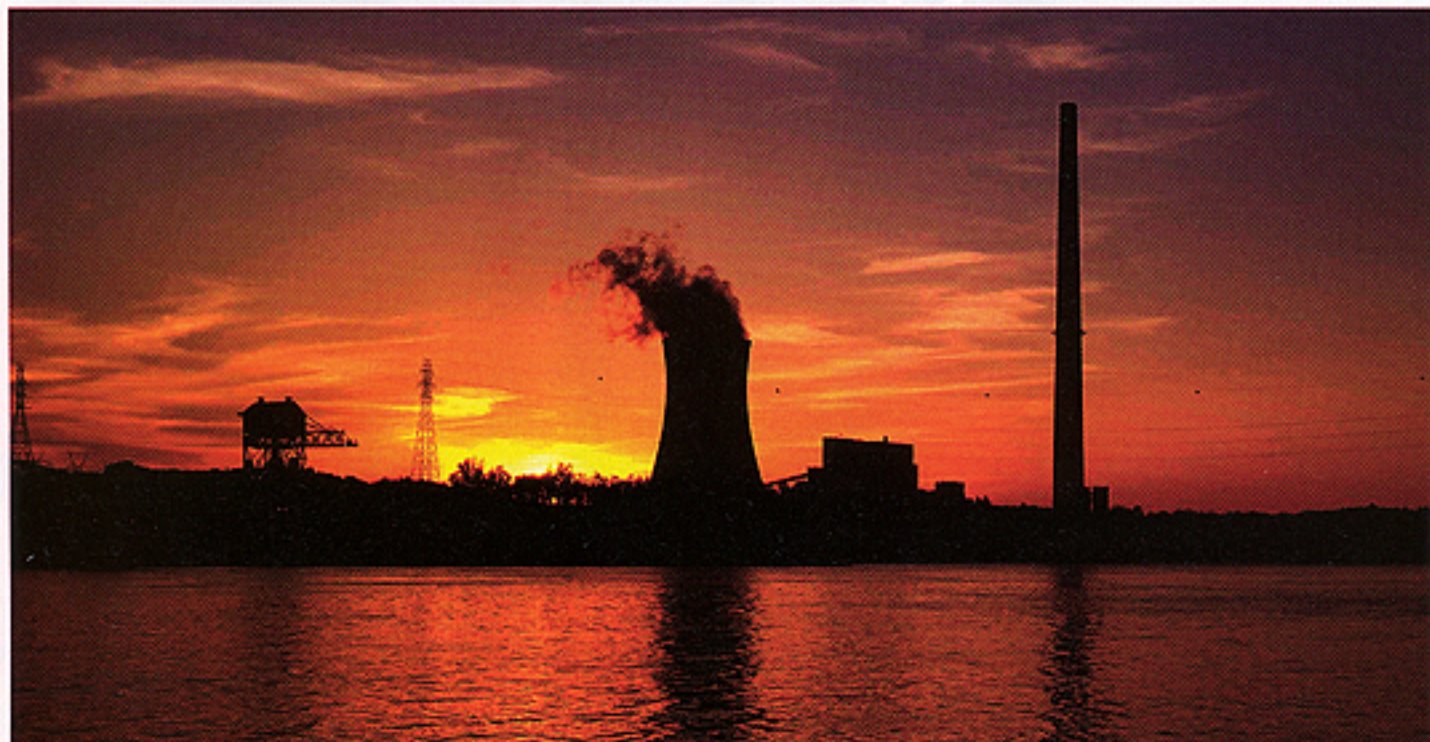
AEP will install a post-combustion carbon capture technology developed by Alstom on its 1,300 MW (electric) Mountaineer Plant in New Haven, W.Va., in 2008. The 30 MW (thermal) product validation will capture up to 100,000 metric tons of CO 2 per year that will be stored in deep saline aquifers at the site. Photo courtesy of AEP.
